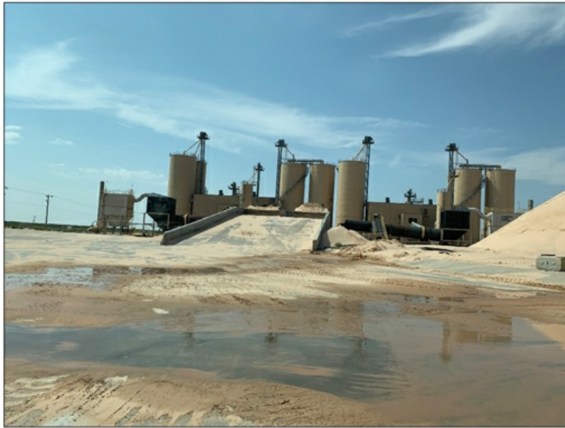
Figure 8.3: Dry Process Plant with Storage Silos
