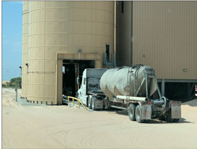
Figure 8.4: Product Loadout Silos with Scales
