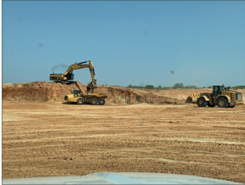
Figure 7.1: Top Bench of Sand Being Removed by Cat 390 Excavator
