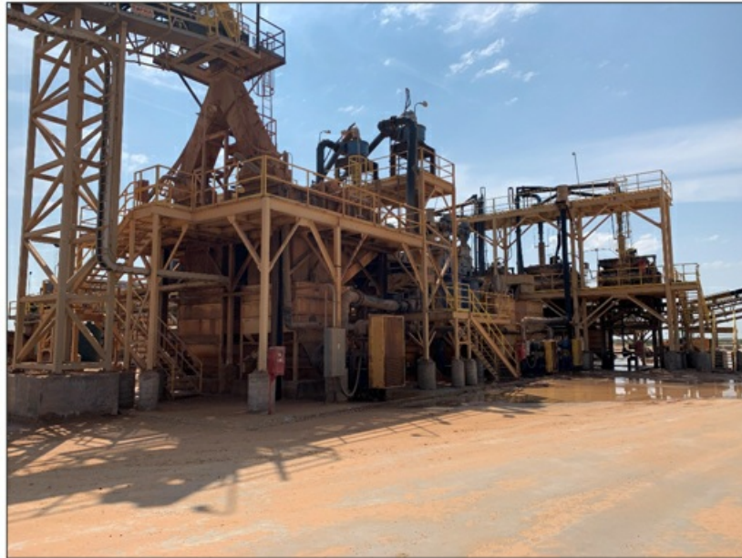
Figure 8.1: Two 300-tph Wet Process Plants in Parallel
